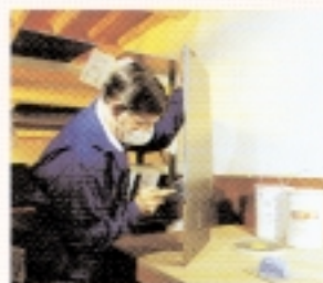
Filling edges of a pre-cut section of Giffab 4109.
