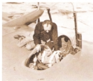
Test pilot instructs Air Force pilot in features of the N9MB control systems. This was a flying scale model of the future XB-35 bomber.
