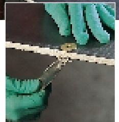
Technician smoothens the edge fill compound and ensures there are no air bubbles along the panel's edges.
