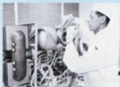
APOLLO environmental control unit is assembled in clean room by Garrett-AirResearch technician. On left are two rectangular lithium hydroxide adsorbers which contain M. C. Gill laminated fiberglass housings.
