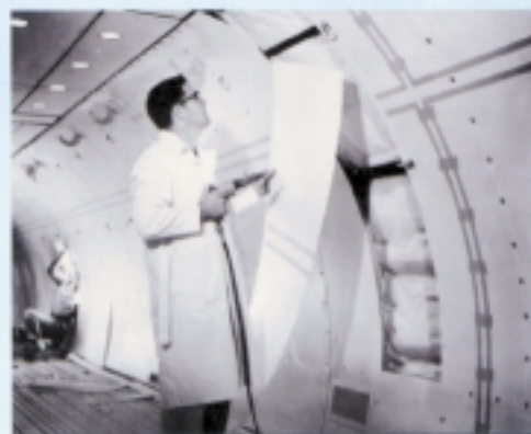
Mechanic installing M.C. Gill cargo liner.
