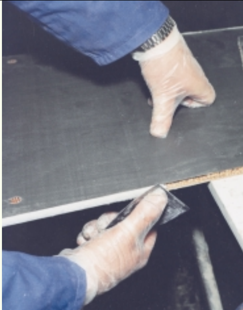
Edge filling the finished floor panel to seal against moisture.
