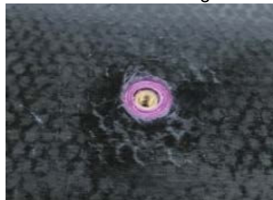
After adhesive cure, check of clean threading
