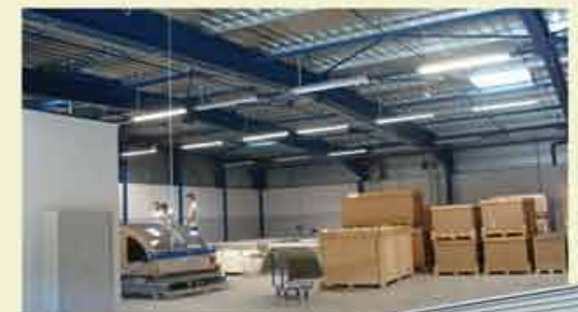
Alcore Brigantine's new building extension.
